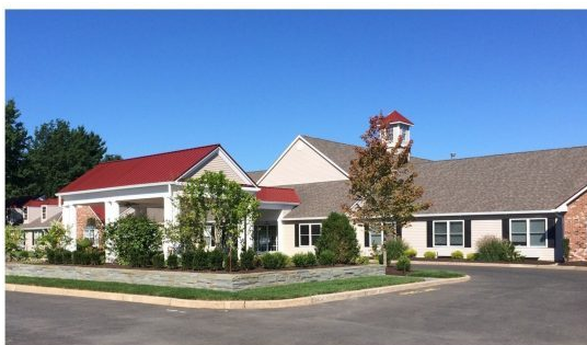
Front View New Entrance with Formal Garden
