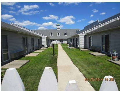
Non-conforming Access & Use
